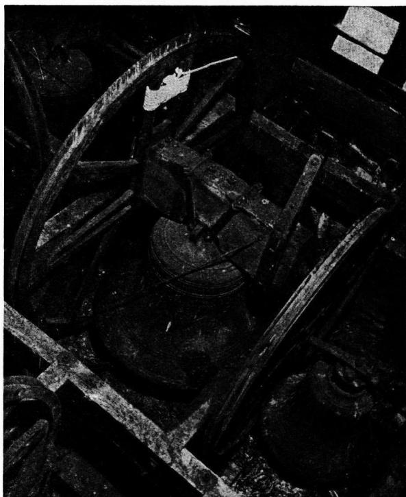
Gawsworth St. James. Belfry before 1955 Restoration.
